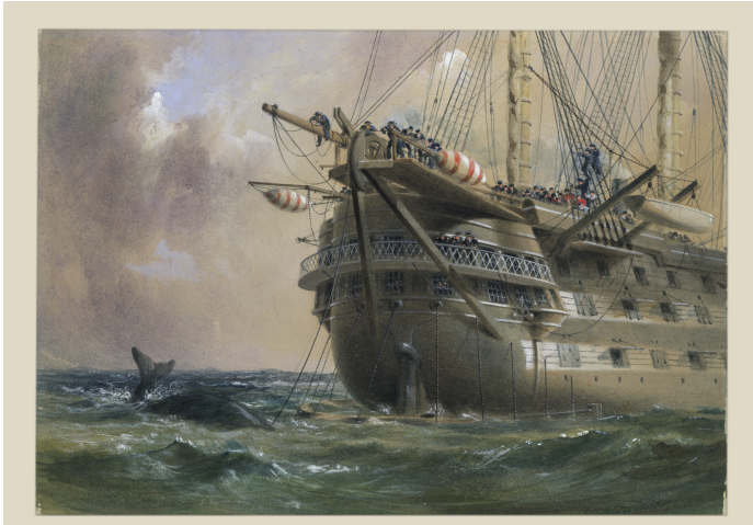
H.M.S. Agamemnon Laying the Atlantic Telegraph Cable in 1858 while a whale crosses the line.
